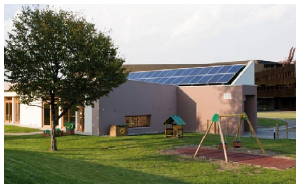
The Company daily nursery in Mogliano Veneto, built according to sustainability standards and endowed with a PV power plant.
