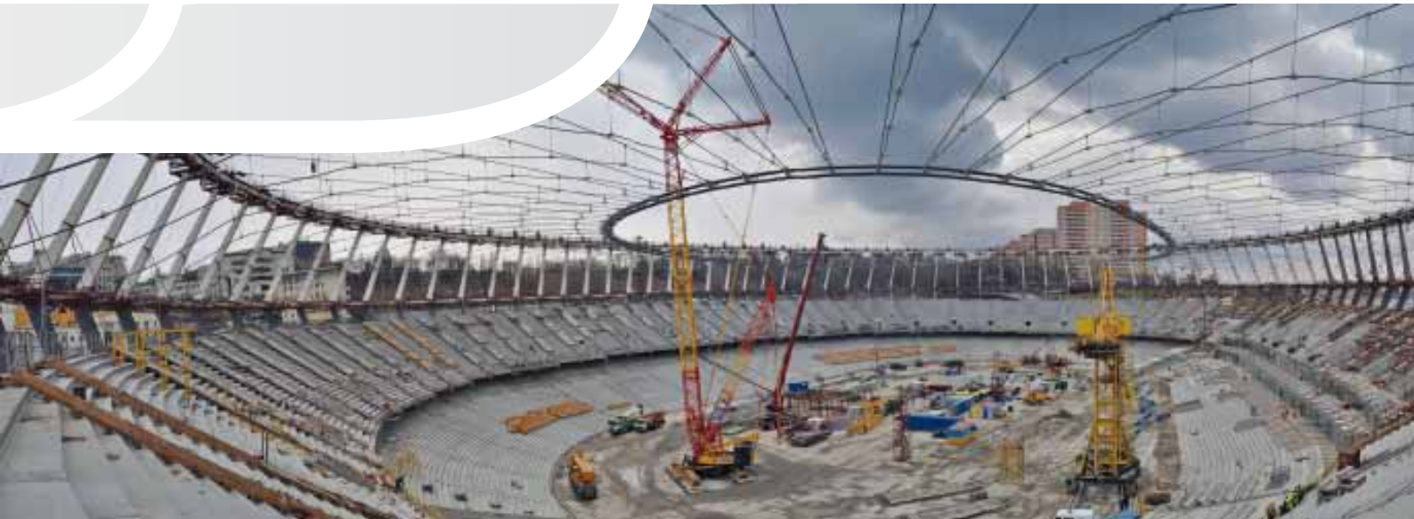
FAGIOLI - Lifting the tensile structure of the new Olympic stadium in Kiev, Ukraine
