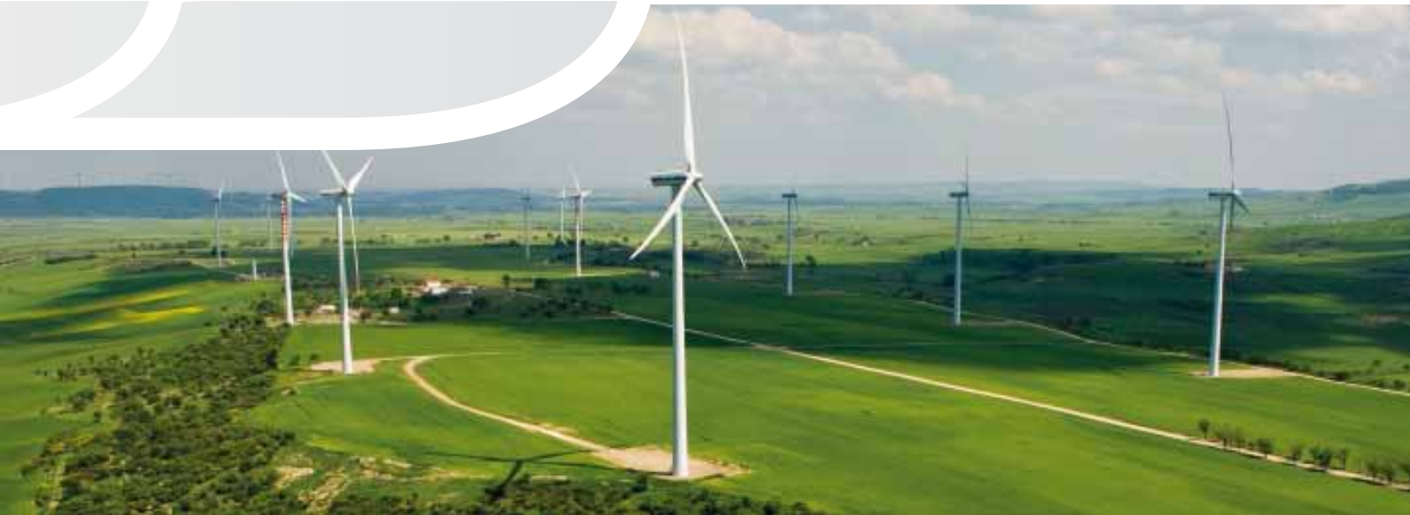
ERG - Troia San Cireo wind farm, Foggia, Italy
