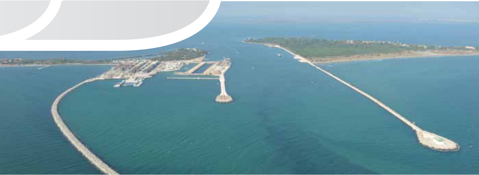
CONSORZIO VENEZIA NUOVA - Mose project, Malamocco port, Venice, Italy
