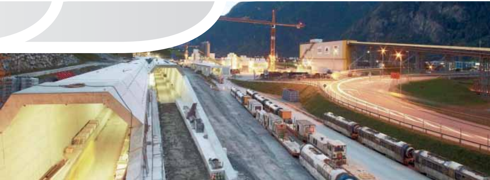
STRABAG - Construction site of Gotthard Base Tunnel, Erstfeld, Switzerland
