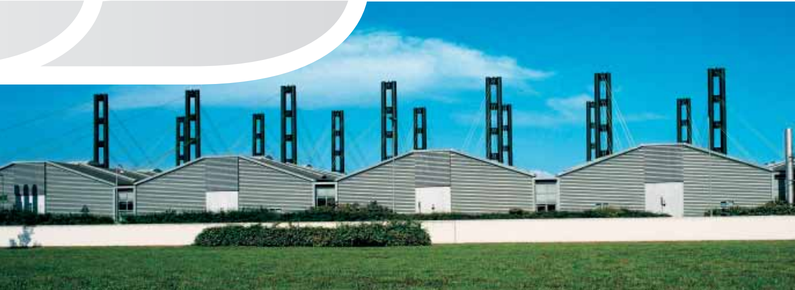
BENETTON – Castrette industrial complex, Villorba, Treviso, Italy
